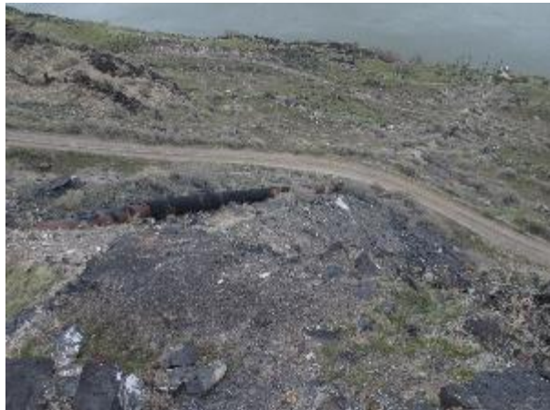
Western Alignment - existing pipeline and pump station from the rim above the project area.
