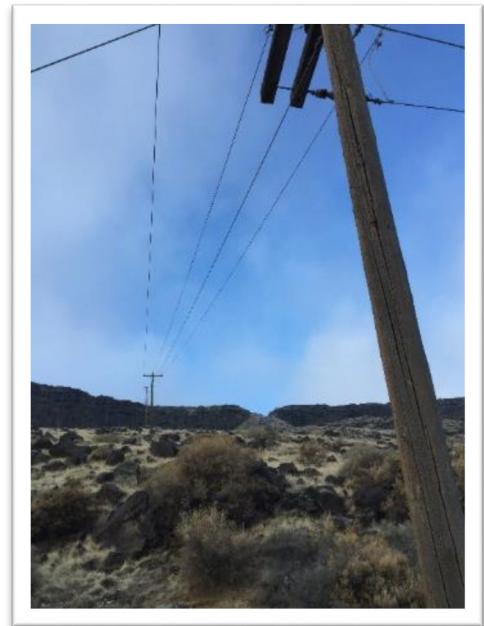
View of Existing Utility Lines and "Notch" at Canyon Rim through Which Existing Simplot Waterline Passes
